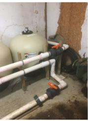
The Equipment Room does not have sufficient space to place this additional filter in line with the existing four, as they go wall to wall with only a couple of inches between. However, along the east wall there is an abandoned pump that could be removed and the fifth filter could potentially fit there. Confirmation of measurements, placement, and measurements should be confirmed prior to undergoing this work.
