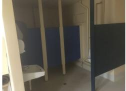
Currently there are two toilets and one sink in each of the washrooms, with one urinal in the male washroom. None of the stalls meet BCBC 2018 requirements for accessible toilet facilities. The sinks also do not meet code requirements for type of fixture, no protection on the piping below the sink, heights of soap and paper towel dispensers, etc.
